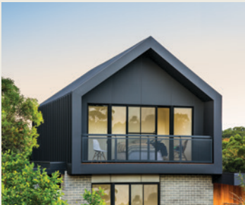
Roof and wall colour: Monument® Matt
